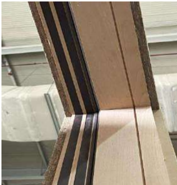
Corner Seal & Intumescent at Door Fame
