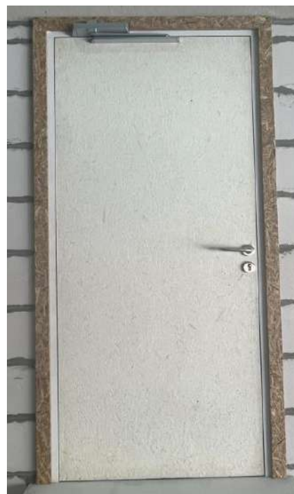
FCC-9000 Flame Core Coat at Door 18 (exposed side)
