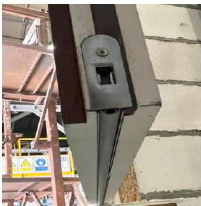
Drop Seal at the Bottom of the Door Leaf
