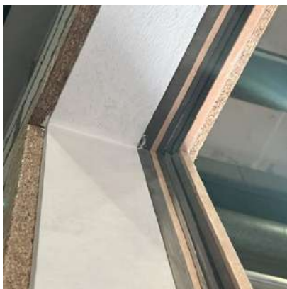
Corner Seal & Intumescent at Door Frame
