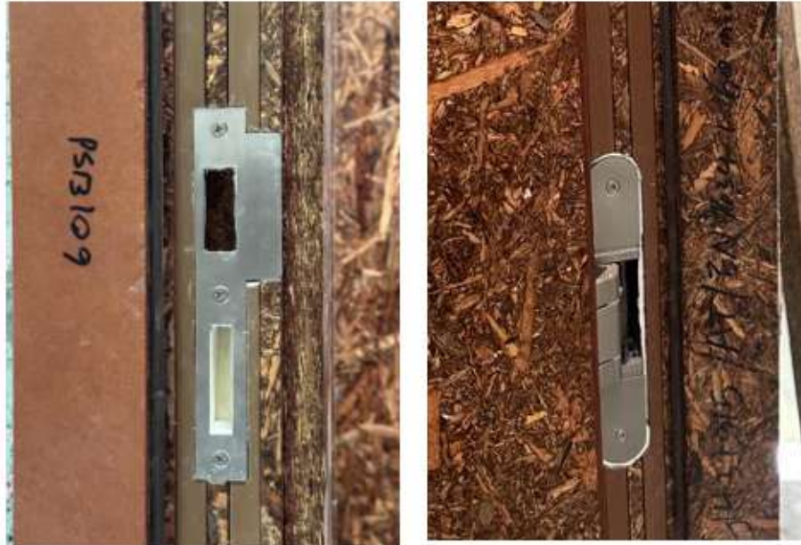
Photo 1. Door frame rebate of door 1 and door 2 respectively.
