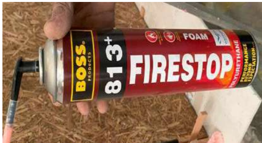
Foam used to fill the gap between supporting construction and frame
