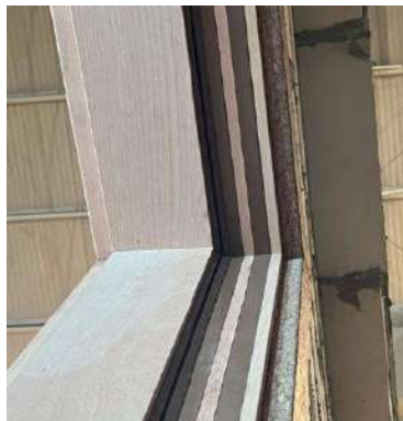
Smoke Seal & Intumescent at Door Frame
