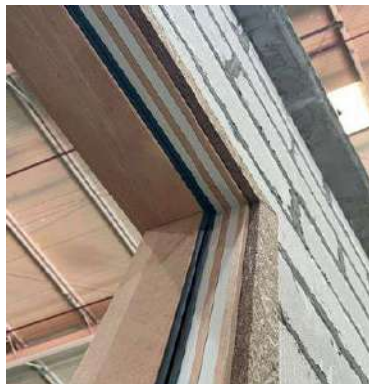
Smoke Seal & Intumescent at Door Frame
