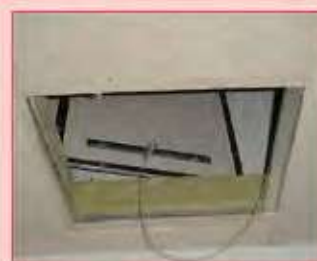
Access panels at fire rated ceiling
