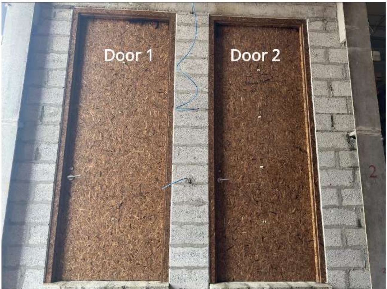
Photo 6. After the Hose Stream Test.
