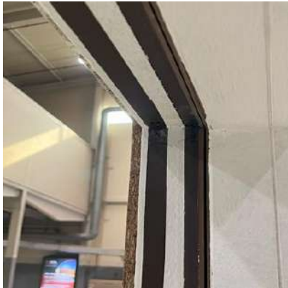
Corner Seal & Intumescent at Door Frame
