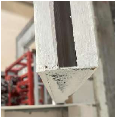
Graphite Liner at the Bottom of the Door Leaf
