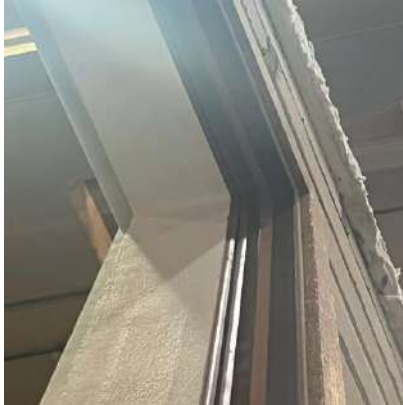
Corner Seal & Intumescent at Door Frame
