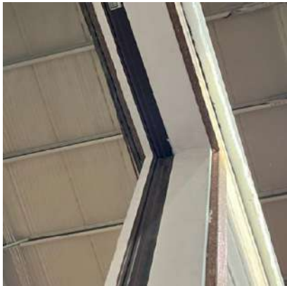
Corner Seal & Intumescent at Door Fane
